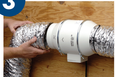
Connect the ducts.
