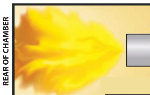
Flame is over-fired
