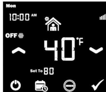
Freeze Protection Off
