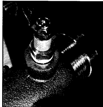
Figure 3 - Installed Low Water Cut Off (LWCO) Probe
