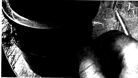
Figure 11 – Installing the Flue Temperature Sensor
