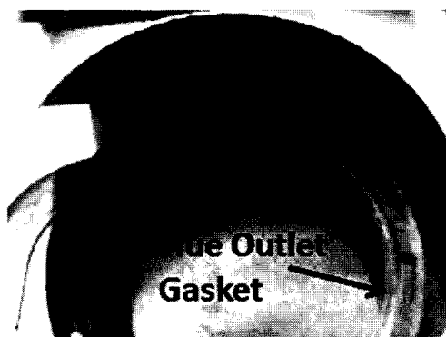
Figure 8 – Exposed Flue Outlet Gasket
