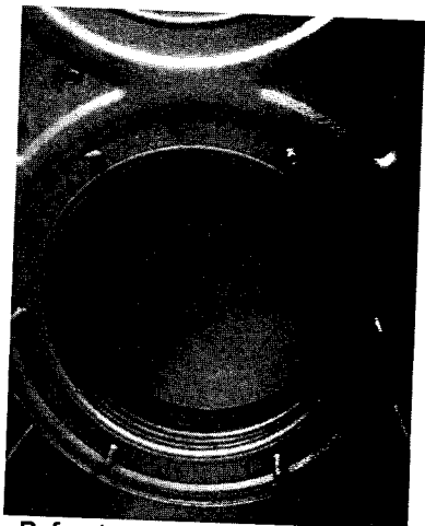
Figure 9 - Refractory Placed in Heat Exchanger
