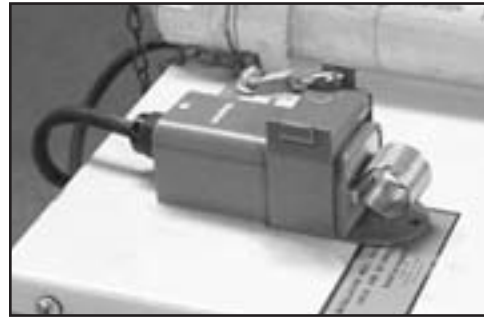
THERMOSTAT LOCK BOXES
