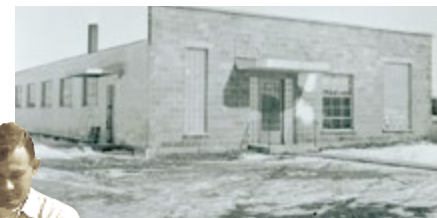
The first factory. 1947
