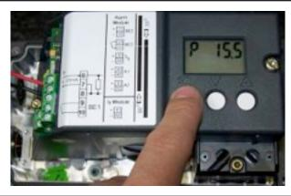
**Step 3:** Once in Configuration mode parameter 1 is displayed in the bottom left hand corner of the positioner screen. Parameter 1 allows the user to select the type of actuator being paired with the device.
